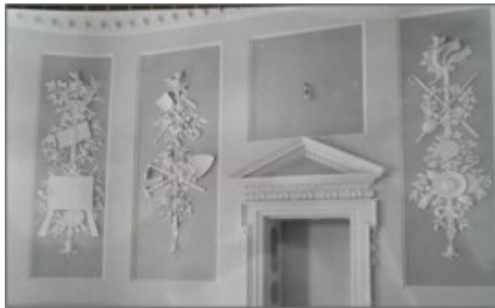
Plasterwork in the drawing-room
