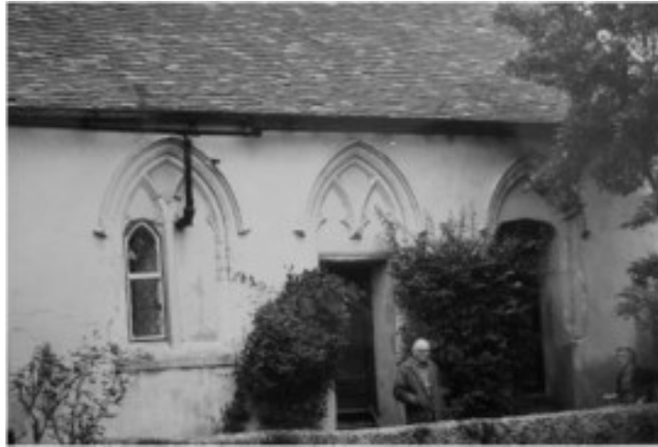
The exterior of the chapel
