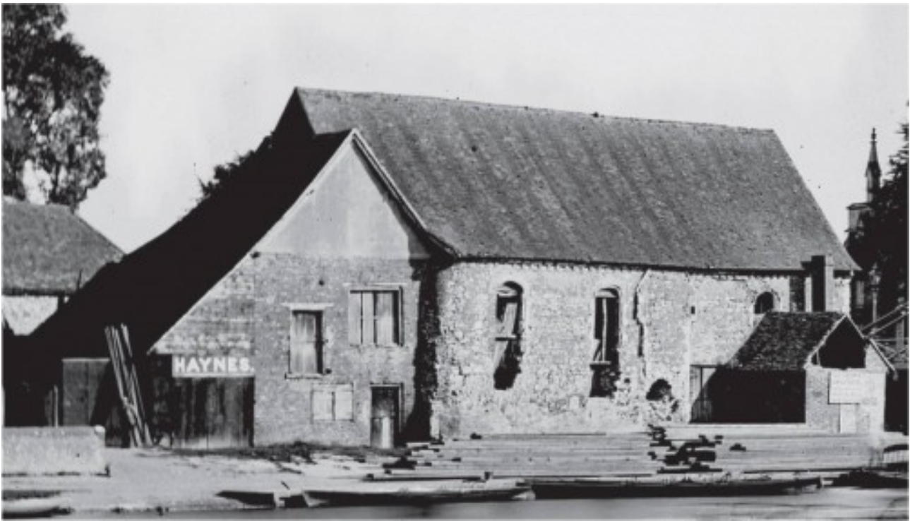
Figure 5 - An enlargement of the Taunt photograph showing the corbel table, window design and the round-headed doorway being unblocked. By permission of Historic England Archive ( select picture to enlarge )
